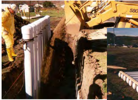
Emitter array in a trench
